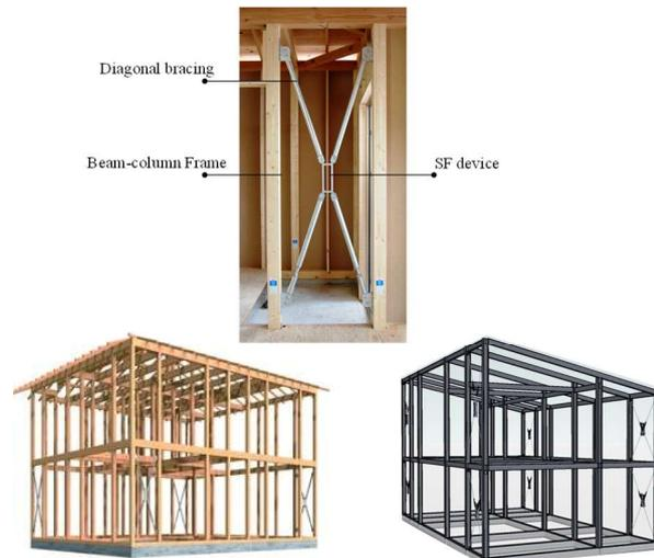
Figure 2: Example of SF structures on wooden frame and steel frame
